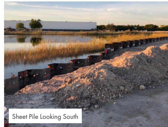
North & East Sides Telecom Duct Bank
