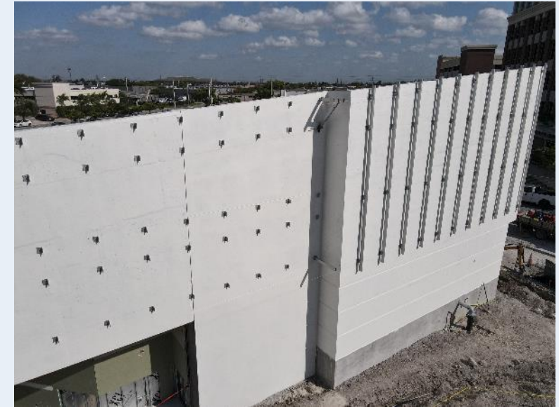
Perforated metal panel support brackets installation March 2022
