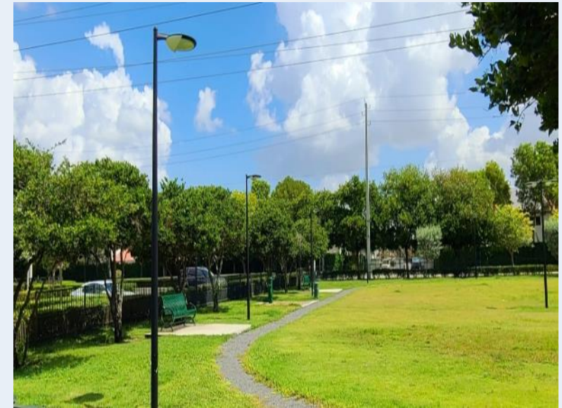
Lights installed June 2022
