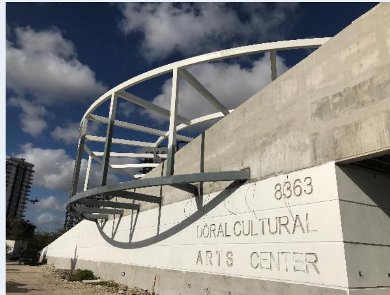
Building Primer Progress South Façade February 2022
