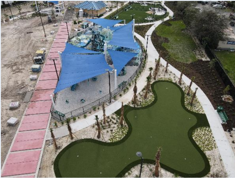
Playground equipment complete January 2022
