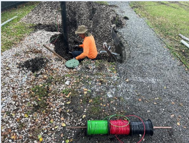
Light Poles Wiring January 2022
