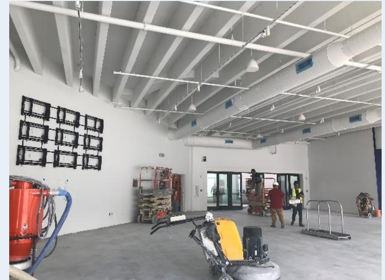
TV wall bracket installation June 2022
