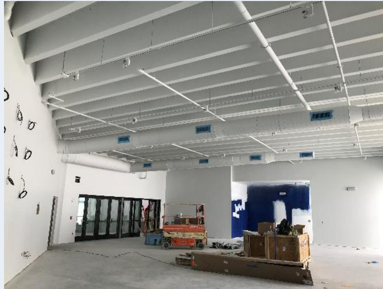
Main art space HVAC ducts and wall finishes progress May 2022
