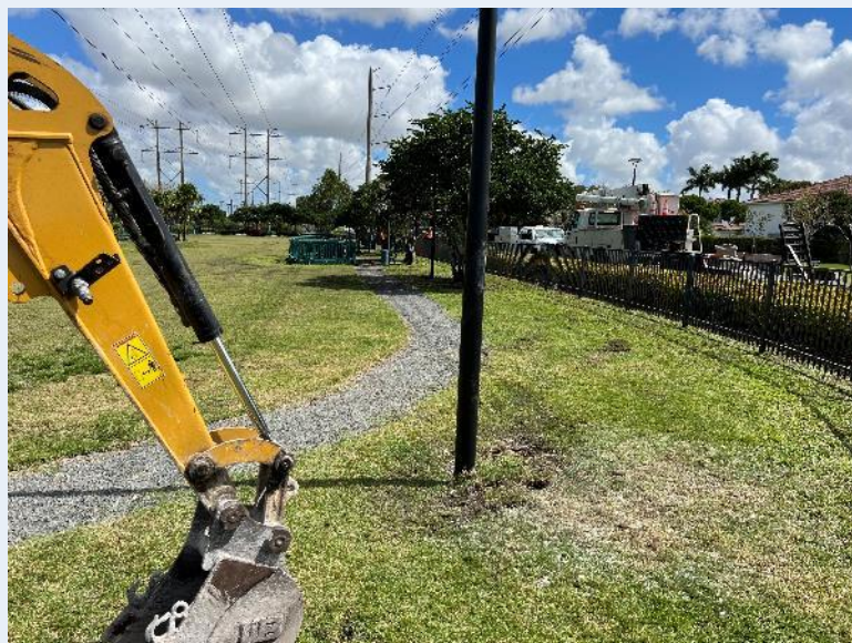
Light pole installation February 2022
