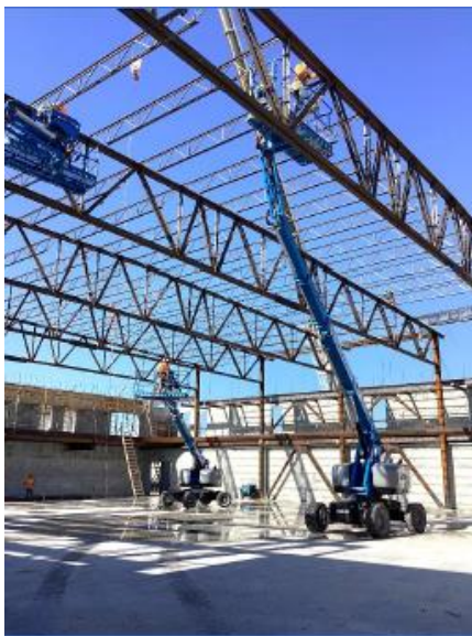
High-Roof at Gymnasium
