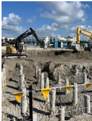
Competition Pool Excavation
