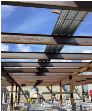
Structural Steel at Rec Center
