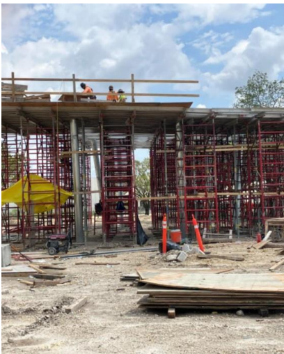
Shade Structure Formwork
