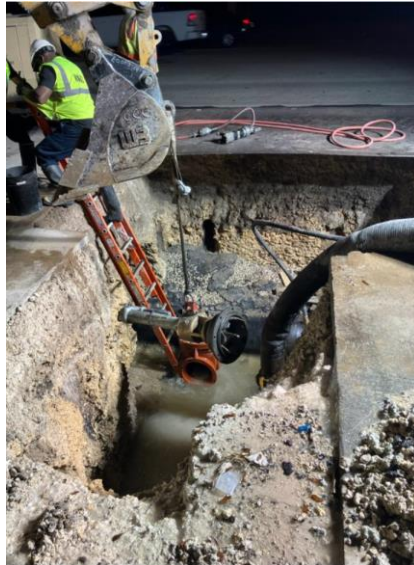
Watermain Tie-in at 87th Ave.
