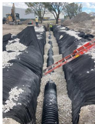
Drainage at Sensory Playground
