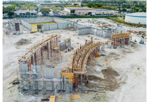
Aerial of Recreation Center Construction
