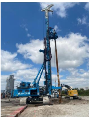
Deep Soil Mixing at Aquatics Facility
