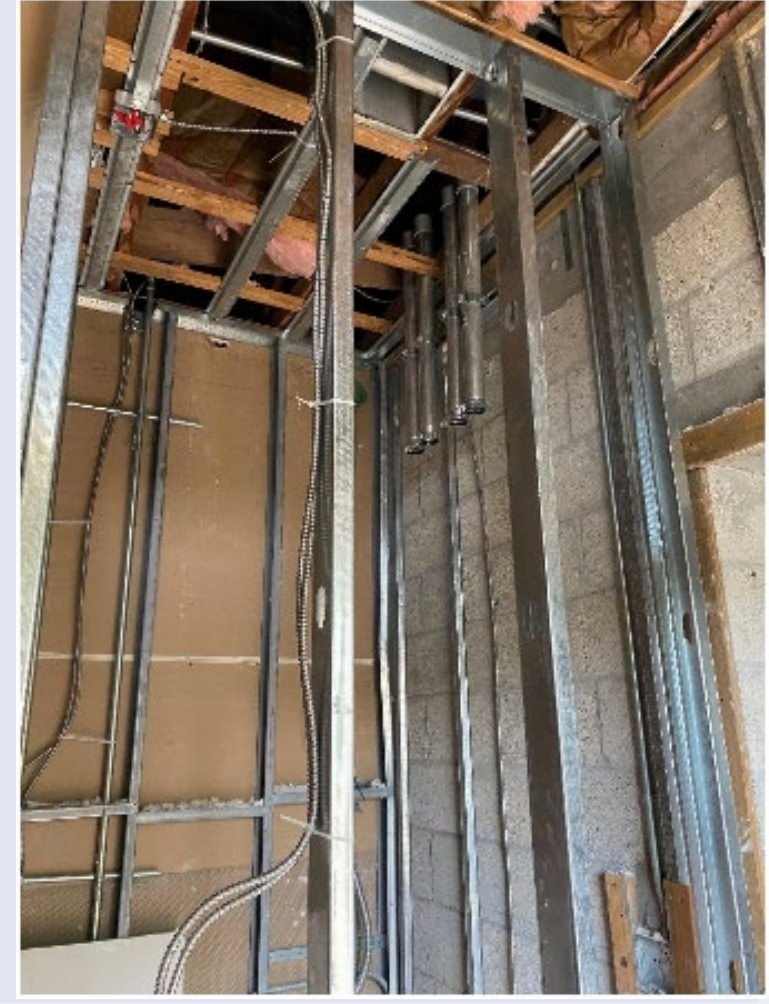
New IT Room being framed out
