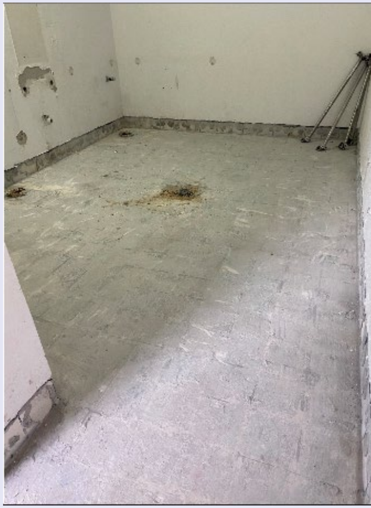
Bathrooms fixtures, floor demo
