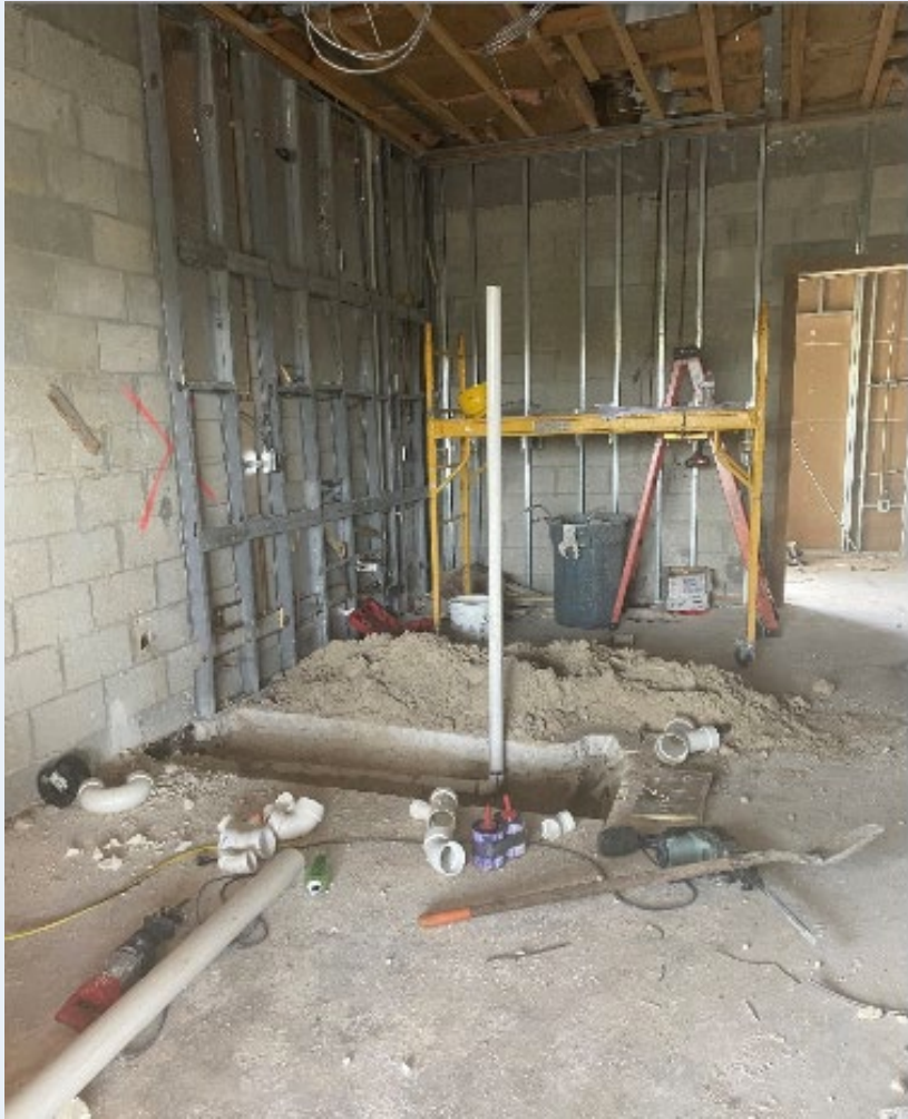
MEP Rough in for New kitchen and HVAC
