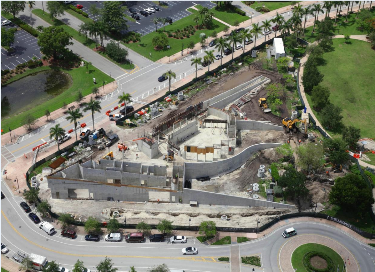
Doral Cultural Arts Center construction progress (July 2021)
