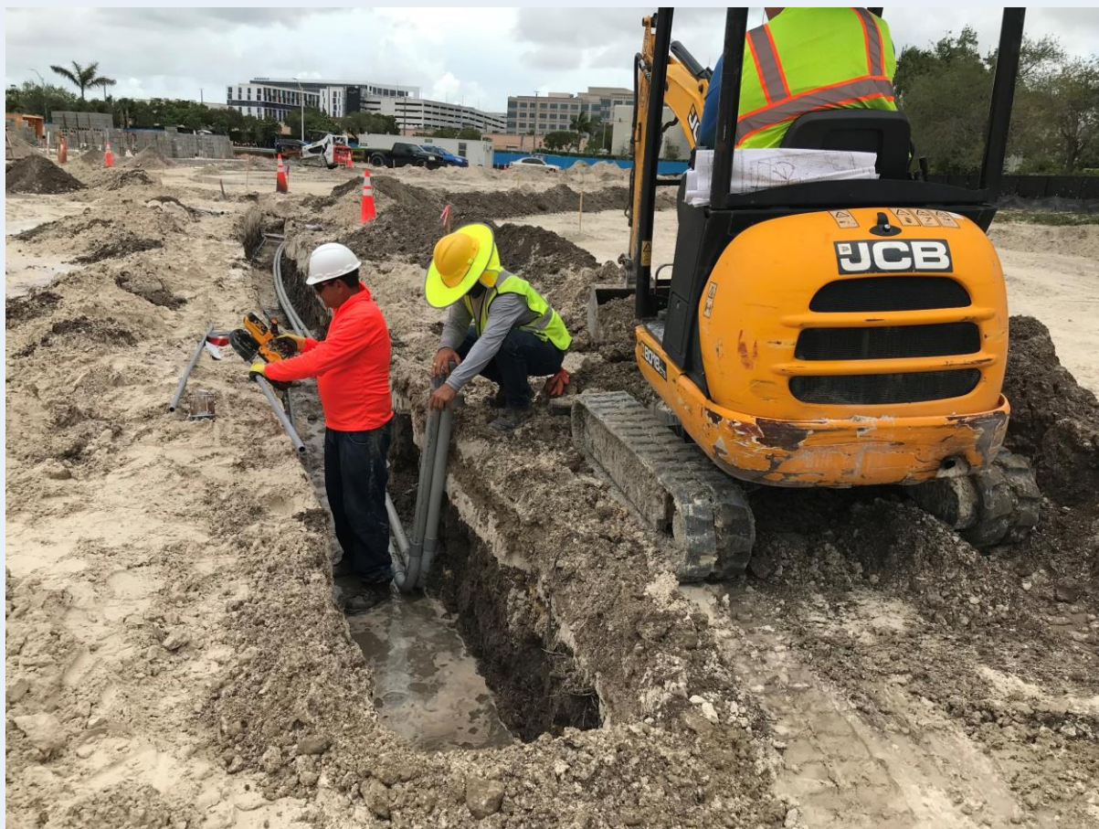
Open trench for the installation of electrical and fiber conduits
