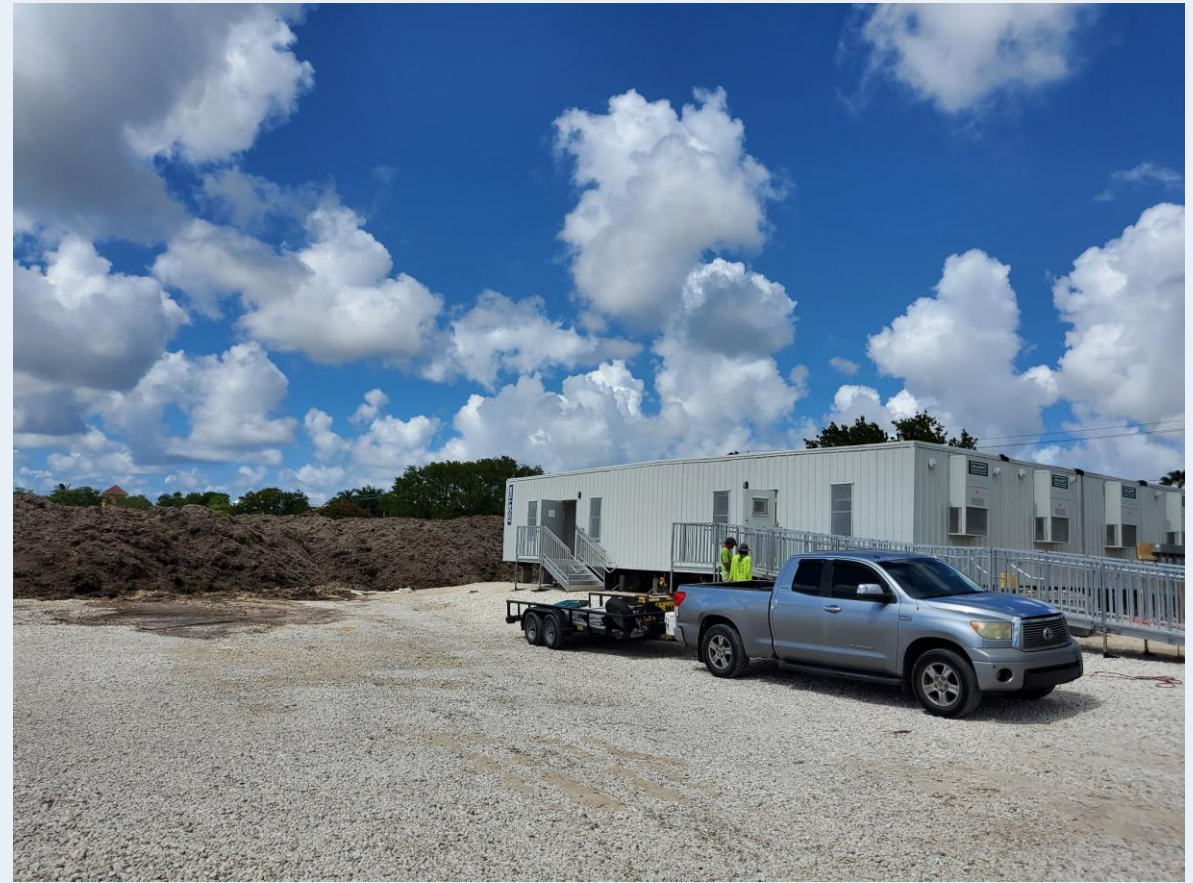
Trailer Installation at Site
