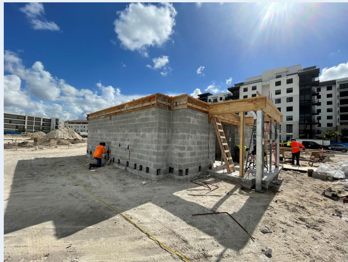
White Course restroom
