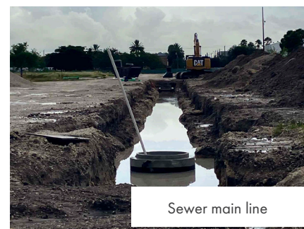
Manhole installation
