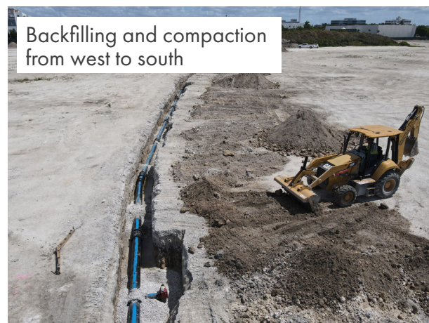
Watermain installation on northside
