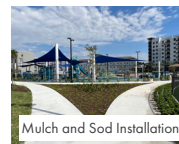
Mulch and Sod Installation
