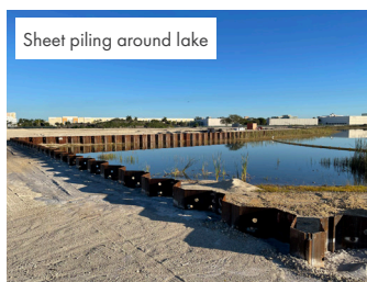
Sheet piling around lake
