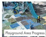
Playground Area Progress
