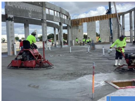
Slab-on-Grade at Recreation Center
