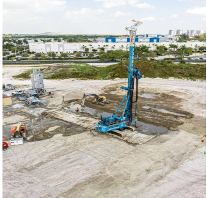
Deep Soil Mixing at Competition Pool
