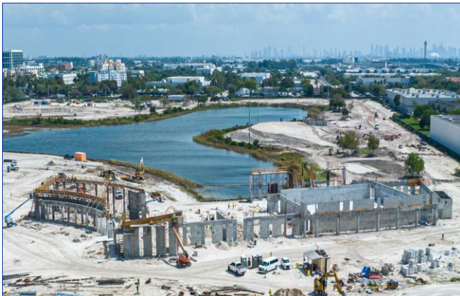
Aerial of Recreation Center Construction
