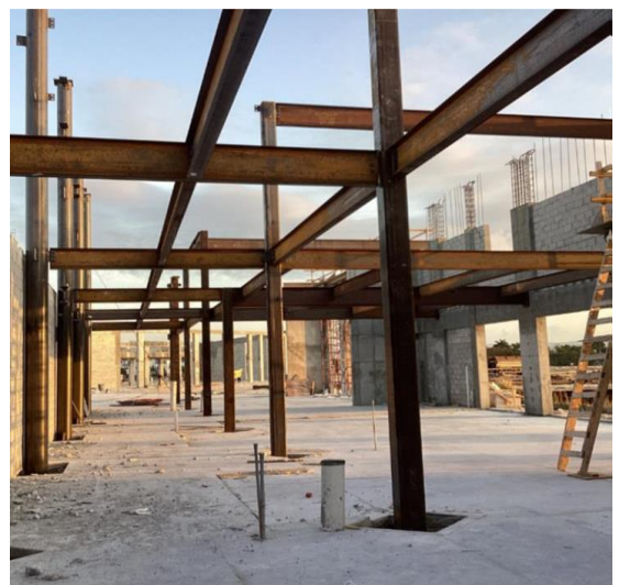
Structural Steel at Rec Center
