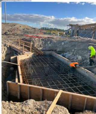
Pedestal Formwork and Rebar for Amphitheater Canopy
