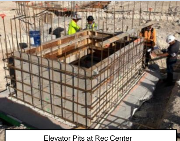
Elevator Pits at Rec Center
