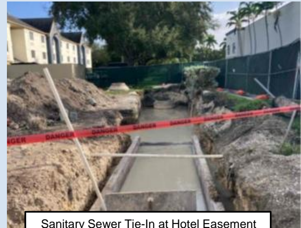
Sanitary Sewer Tie-In at Hotel Easement
