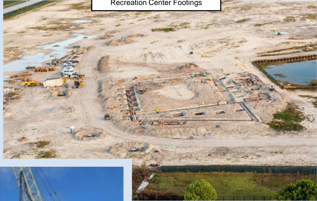
Recreation Center Footings
