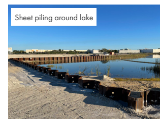
Sheet piling around lake
