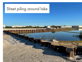
Sheet piling around lake
