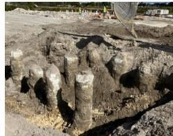
Excavation of Piles at Amphitheater
