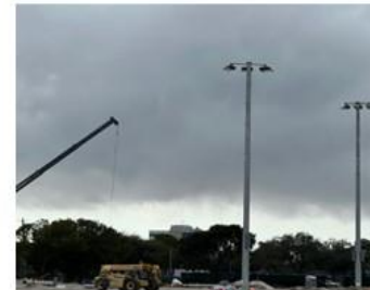
Sports Lighting at Skatepark with Pump Track
