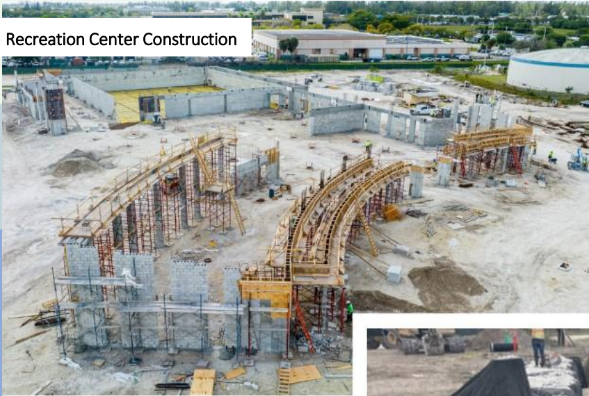
Columns and Beams at Recreation Center
