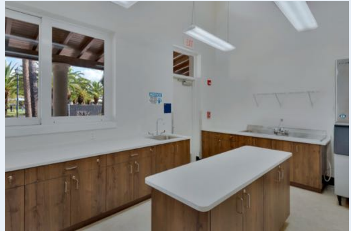
Modernization of kitchen with new millwork and flooring
