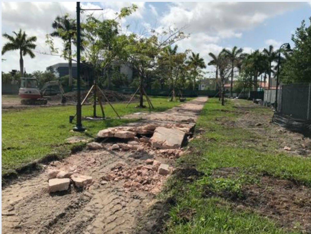
Contractor demolishing existing sidewalk as part site clearing Activities.
