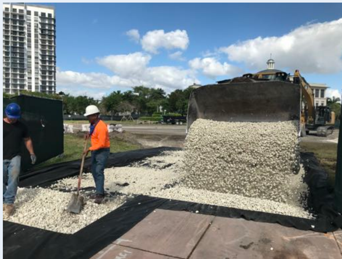
Contractor preparing gravel truck entrance into the site
