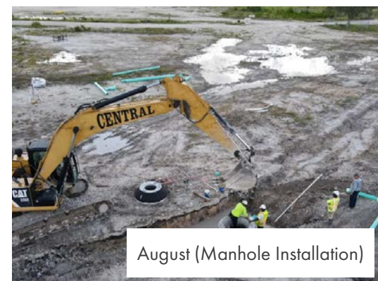
August (Sanitary Sewer Main Line and Laterals by Aquatics Facility)
